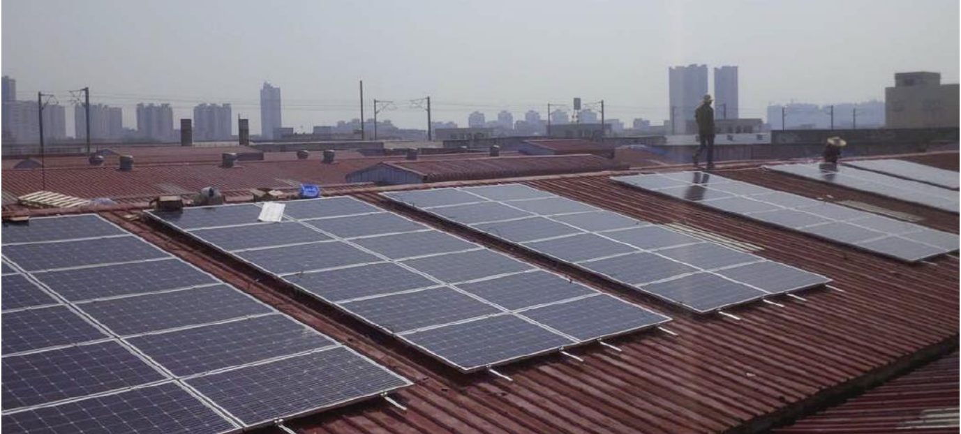
Photo: Solar panel installation at final assembly supplier in China
